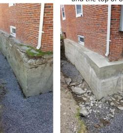
rebuilt. The "new" foundation (around the extension building) was still in good shape.
