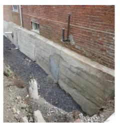
After preparing the drainage ditch for laying the eventual drainage pipes, the next step was sealing the foundation . . . which involved a
